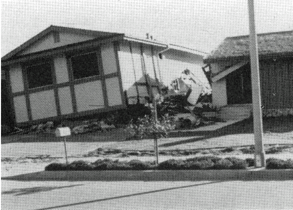
Building has collapsed, partially collapsed, or moved off its foundation. Condition: UNSAFE
